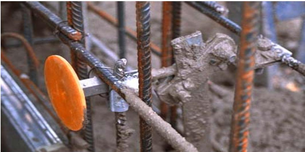
Fig 3:Equipotential bonding connector during building phase (Obo Bettermann)
