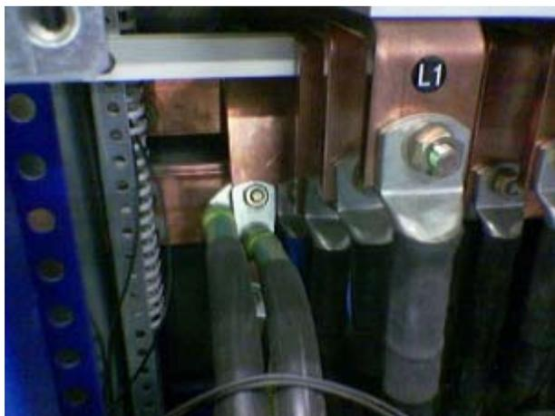
Fig 7: TN-S: Bridge between 3 transformers
